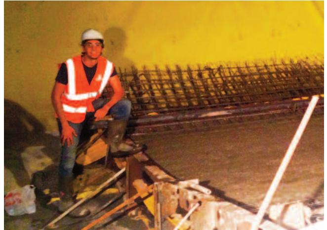
The construction process starts with a jackhammer, which breaks the hard surface. Shotcrete is then applied on the surface of the excavation and the required number of bolts are driven in so that the tunnel is connected to the main land layer. Bolts are required to carry the tunnel by applying tension.
